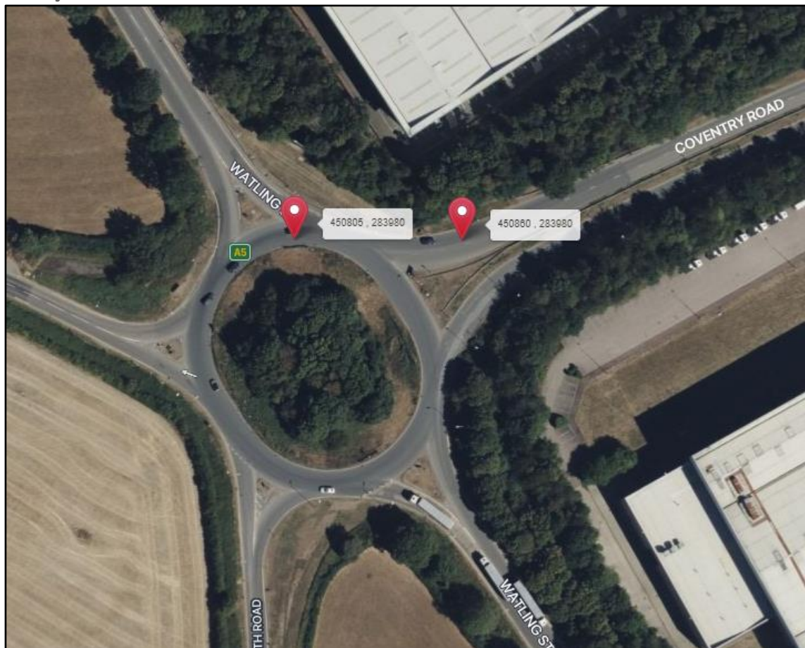
Figure 2.7: Cross in Hand Roundabout (A5 Watling Street/A4303/B4027/Coal Pit Lane) Road junction
