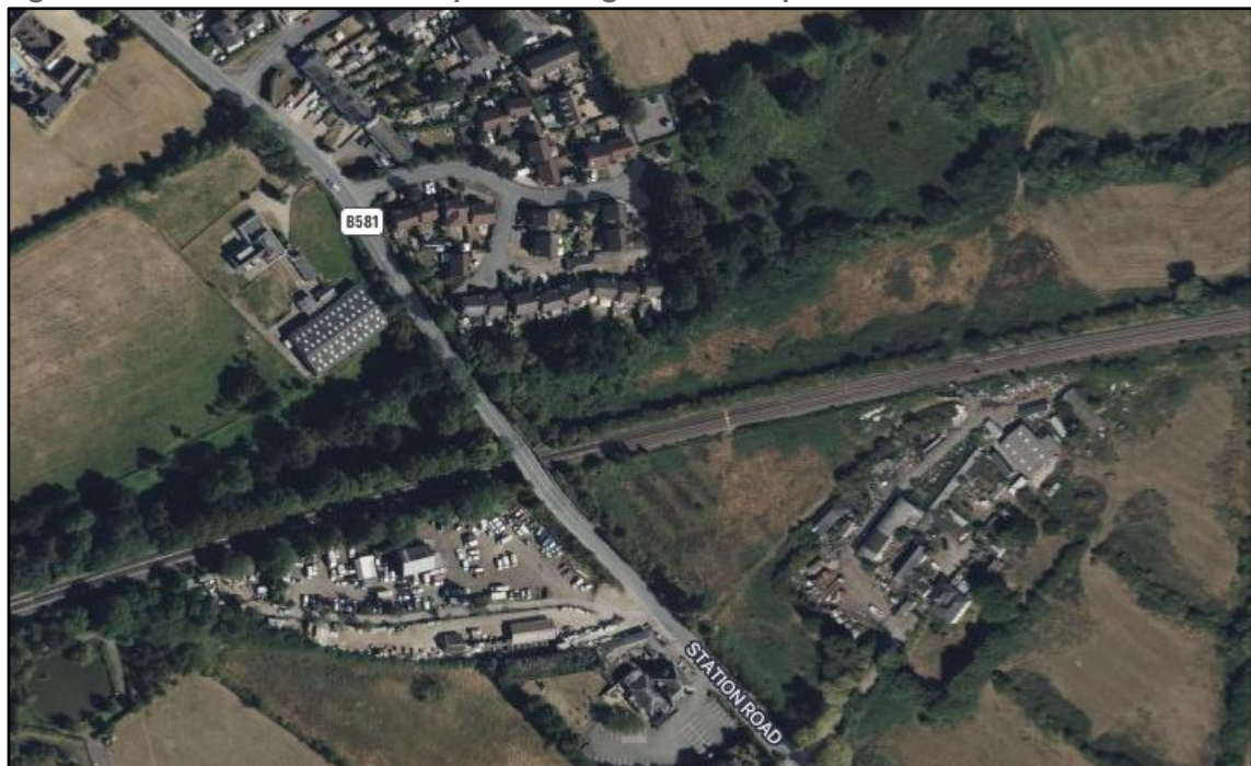
Figure 2.12. Station Road Railway Overbridge Elmesthorpe
